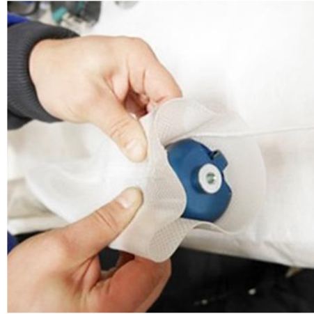
3. Make folds to the Silicone bladder and tape it to the Packer
