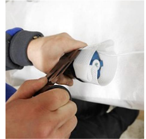
3. Make folds to the Silicone bladder and tape it to the Packer
