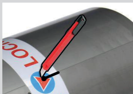
Cutting halfway through the adhesive strip
