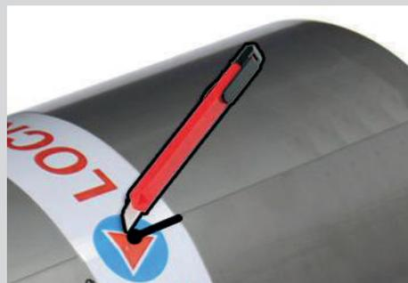
Cut the adhesive tape half-way through
